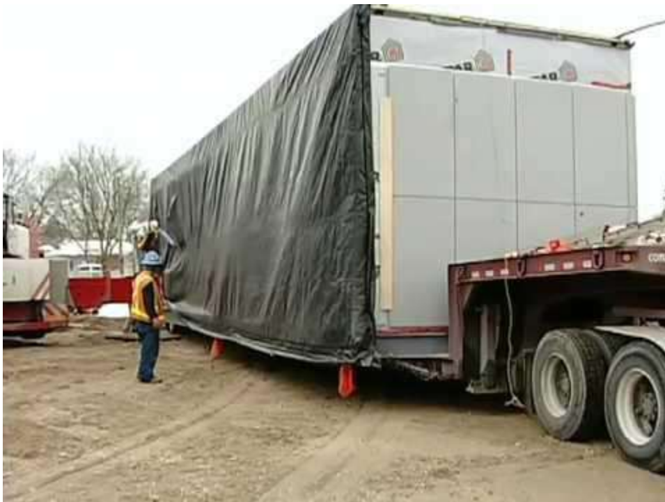
Picture of modular structure ready for transport
